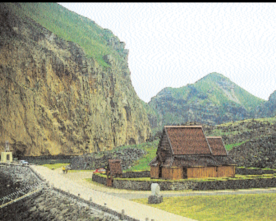
▲ CHURCH ON A VOLCANIC ISLAND: Although the replica of the Haltdalen Stave Church stands on a weather-beaten outpost at the approach to Heimaey in the Vestmanna archipelago on Iceland, it is well protected from the raging wind and waves by a wall of hardened lava. To be on the safe side, a gallery was added to reinforce the outside perimeter of the church.
