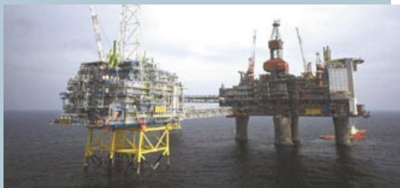
UNIQUE: Statoil has stored two million tonnes of CO 2 under the ocean floor of the North Sea’s Sleipner field since October 1996. The project is currently the only one of its kind. (Photo: Statoil)
